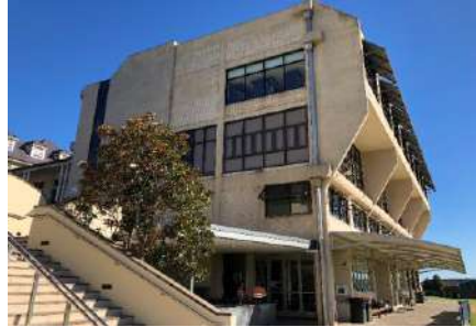
View of TSC Stevenson Library, Scots College. Showing southern facade of building. Looking north. Inspected 11.03.2018
