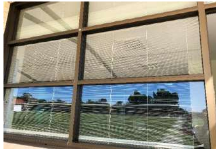
View of TSC Stevenson Library, Scots College. Showing typical aluminium windows throughout building. Inspected 11.03.2018
