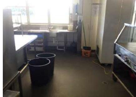
View of: kitchen area Inspected on 11.03.2018
