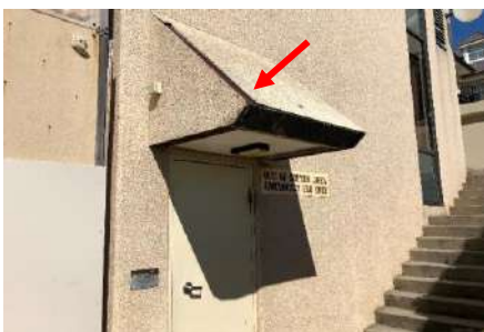
View of TSC Stevenson Library, Scots College. Showing Sample AS1 location . Fibre-plaster material awning above emergency exit along northern facade.
