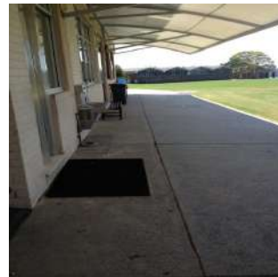
View of: outside of building Inspected on 11.03.2018
