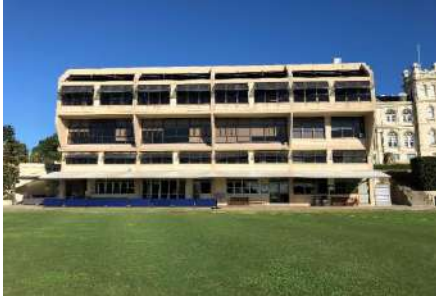
View of TSC Stevenson Library, Scots College. Showing eastern facade of building.
