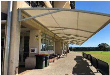
View of TSC Stevenson Library, Scots College. Showing eastern aluminium awning. Looking north. Inspected 11.03.2018
