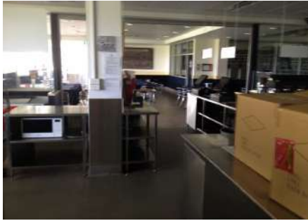
View of: kitchen area Inspected on 11.03.2018
