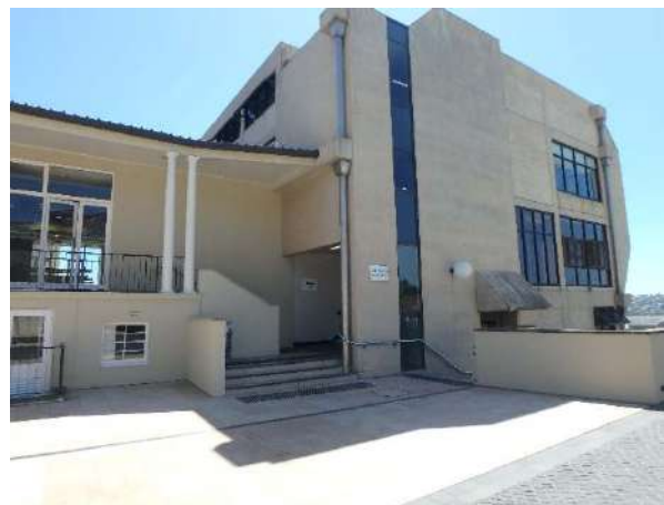
Figure 27. Southern end of Stevenson Library, and adjacent Dining Hall from Quadrangle
