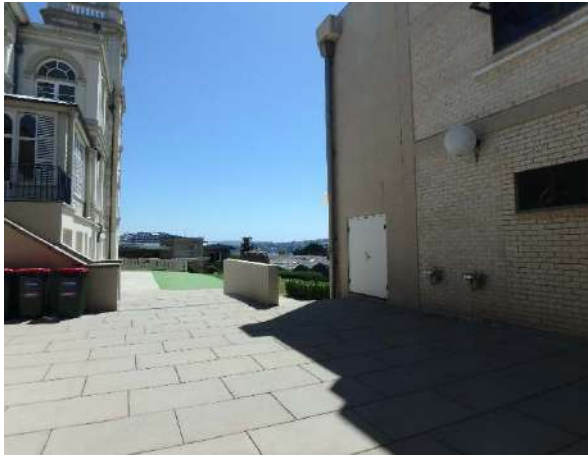
Figure 28. Courtyard behind Stevenson Library (right), with Aspinall House on left
