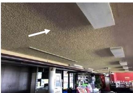
View of TSC Stevenson Library, Scots College. Showing Vermiculite ceiling above Library reception area. As per Sample AS4 location. Inspected 11.03.2018
